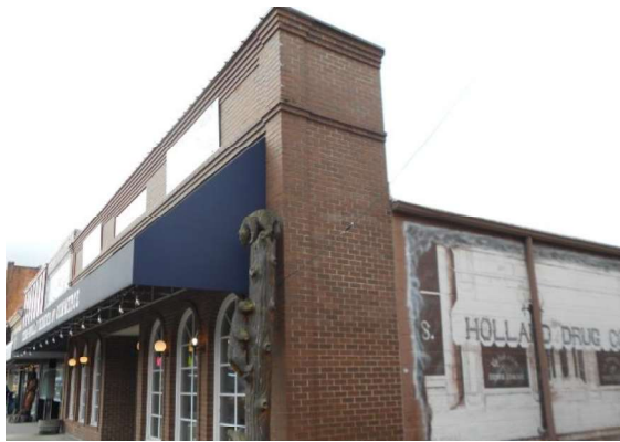
A false front disguises the rest of this single-story building, creating a more impressive, eye-catching façade.
