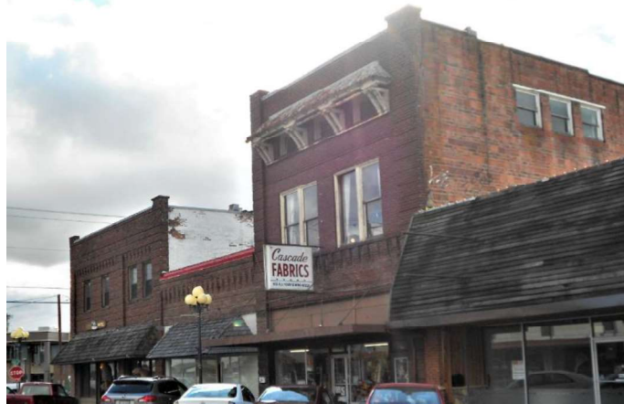
Examples of historic Art Nouveau style architecture in downtown Sedro-Woolley displaying tall, decorative fronts.
