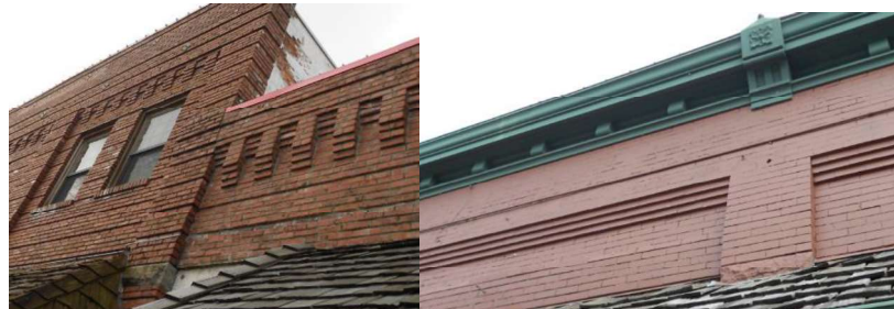
Examples of remnant dentil detailing (left) and crown molding (right) in Sedro-Woolley’s CBD.
