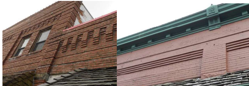
Examples of remnant dentil detailing (left) and crown molding (right) in Sedro-Woolley’s CBD.
